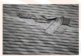
asphalt shingles, deformed edges, curled or missing shingles, missing or loose tabs, loose/slipped or missing slates/roof tiles, growth of moss and lichen which could signal the underside of the roof is decaying
