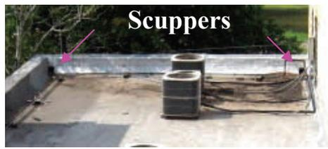
Scupper can easily become blocked by a combination of leaves and twigs. Then ice may build and block the scupper completely.
