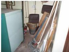
When a boiler room becomes the storage area, routine visual examination and servicing of the equipment is in serious doubt. Boilers and their supporting machinery, controls, piping and valves need to be checked and maintained regularly. If you can't get to the equipment, how is that being done?
