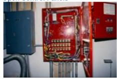
A key indication that something may not be quite right is to see any of the following: an open boiler control panel; a boiler access panel removed; an electrical junction box cover missing; or boiler circuit wiring in disarray.
